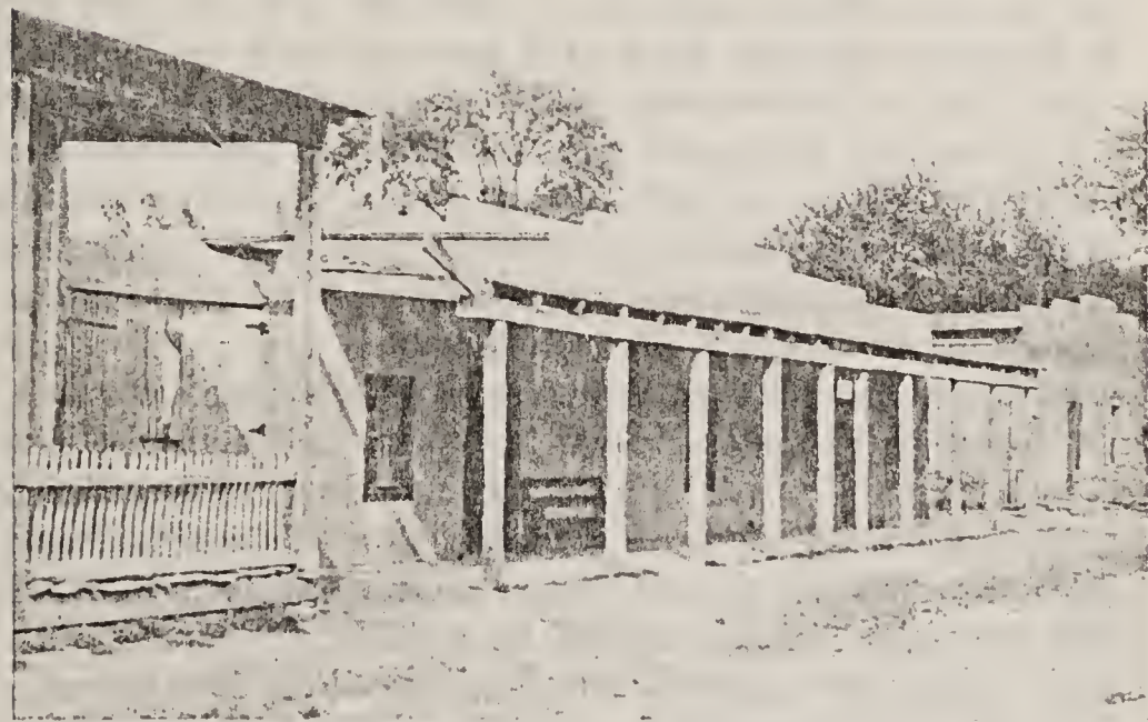
Upper, Ruins of the homestead of Colonel King S. Woolsey, near Agua Caliente, Arizona. From the tree shown near the ruins, eight bad men were hanged at one time by Woolsey and his neighbors in a general clean-up. Lower, the home of Kit Carson, Taos, New Mexico. The building is in the same condition as at the time Carson lived in it
